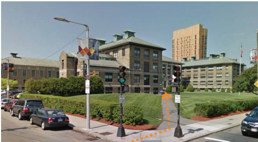
View: from Ruggles St./Parker St. looking towards entry
