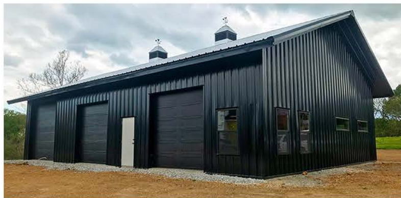
Pre-fabricated metal barn
